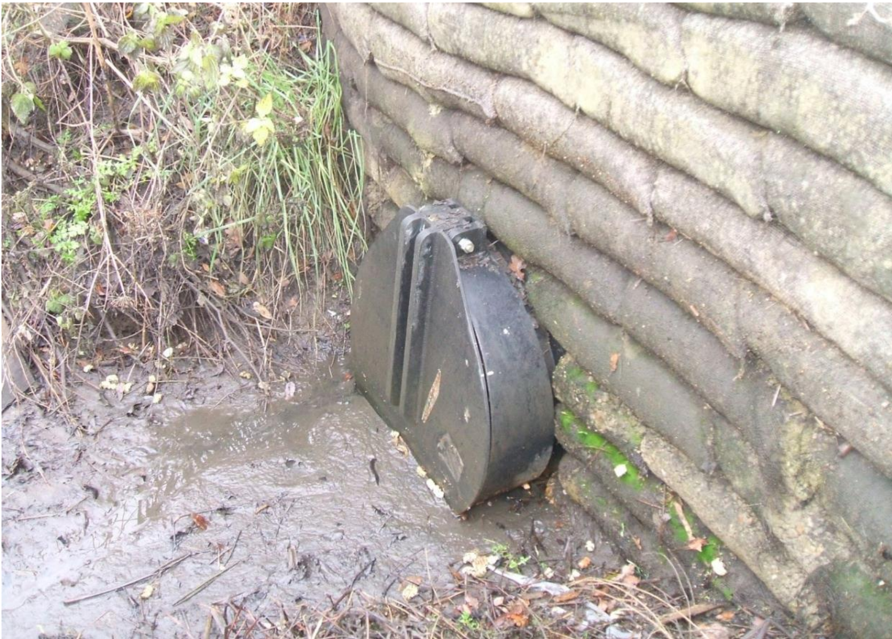
Working Flap Valve South of Lakeside Road (2009)
