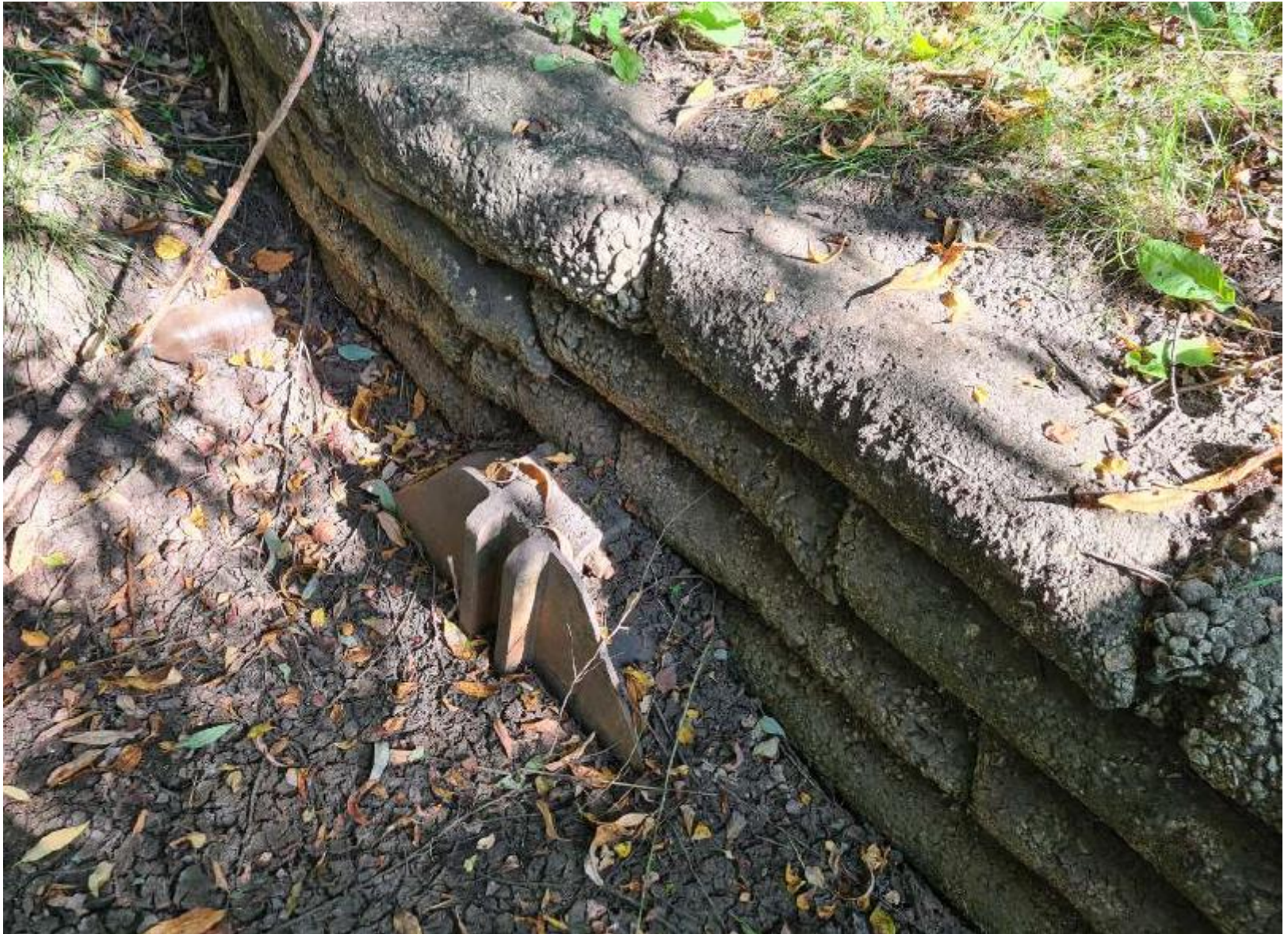
Silted Flap Valve (2020) serving a 300mm pipe flowing into the Blackwater River
